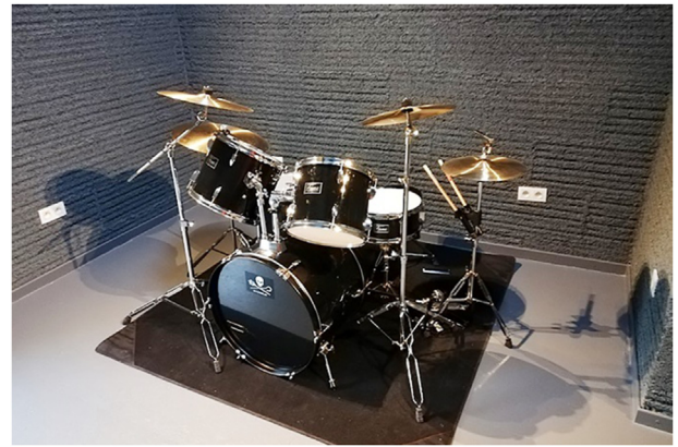
Figure 8. Sound studio with hempcrete [193].
