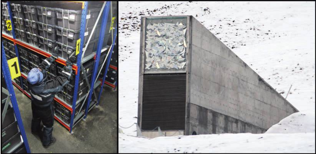
FIGURE 17.3 The Svalbard Global Seed Vault, a secure seed collection in an abandoned coal mine on the Norwegian island of Spitsbergen in the remote Arctic, providing a continuously frozen environment. Seeds of crops are stored at -18^{\circ}\text{C} , and if the electrical supply fails, the permafrost keeps temperatures at no higher than -3.5^{\circ}\text{C} . Almost 900,000 seed samples of more than 5000 different species have been deposited. The facility is expected to grow to become the world’s largest collection of seeds of crops, with a capacity to store about five million samples. Known as “the doomsday vault,” the purpose is to back up important crop germplasm in other seedbanks that could be destroyed by disaster. Unlike conventional seed banks that exchange seeds with numerous individuals and other institutions, only the depositor seed banks have access to their materials. Left: Containers of seeds stored on shelves. Public domain photo by NordGen/Dag Terje Filip Endresen. Right: Entrance. Photo by Bjoertvedt (CC BY 3.0).
